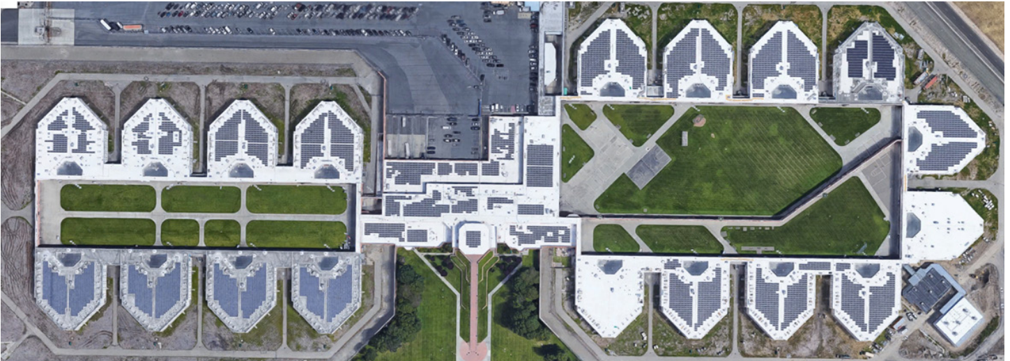
Figure 2. (Imagery, Google), aerial view of the facility, showing the PV roof array
