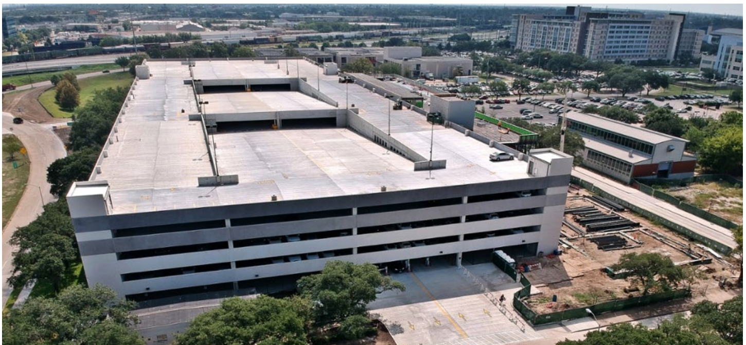
Figure 11. Garage 5: Elgin st. Garage ( https://www.uh.edu )
